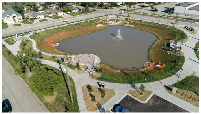
The District partnered with the Village of Niles to construct a relief storm sewer and surface and underground stormwater storage areas near Greenwood Avenue to provide flood relief to nearby homes and businesses. The project has the capacity to store and detain more than 4.5 million gallons of stormwater to help mitigate flooding in Niles.
