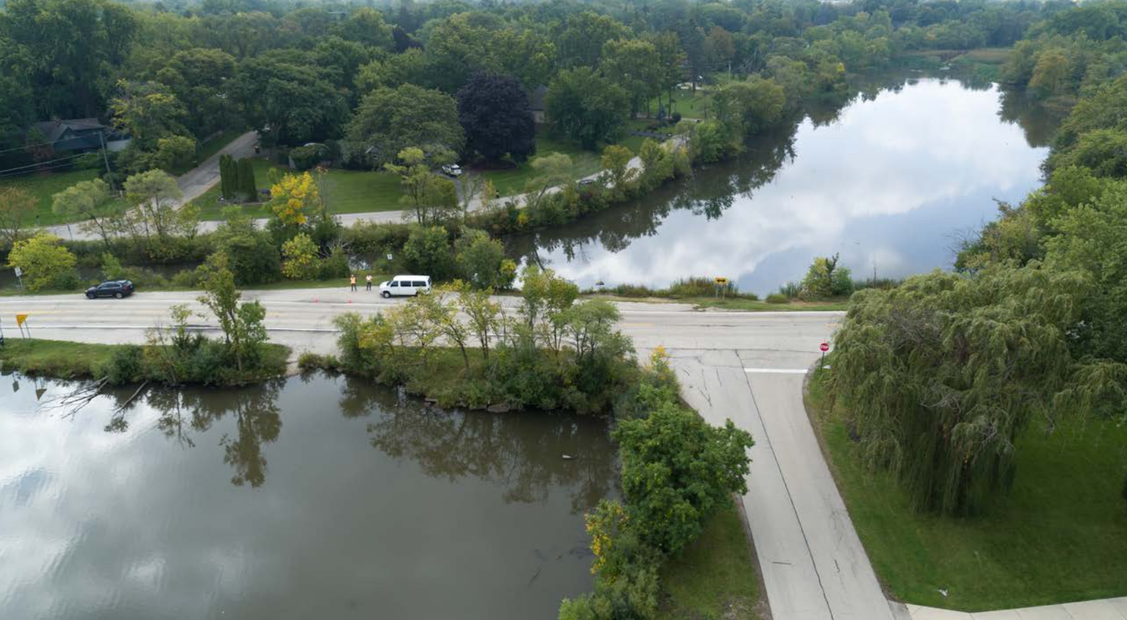
The Willow Road Flood Control Project is designed to provide relief for Prospect Heights residents who have not been able to enter or exit their homes on rainy days.
