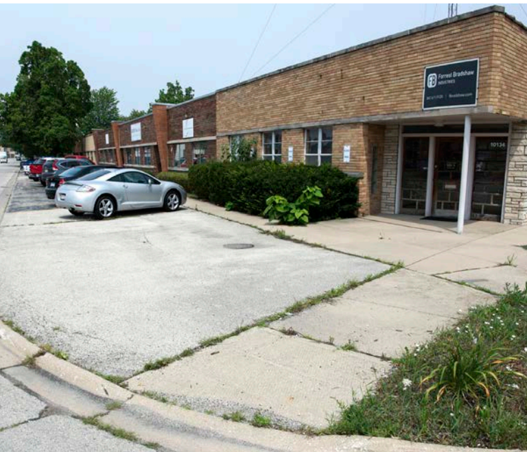
LEFT: The corner of Sarah Street and Pacific Avenue in Franklin Park before completion of the MWRD's GI project.
