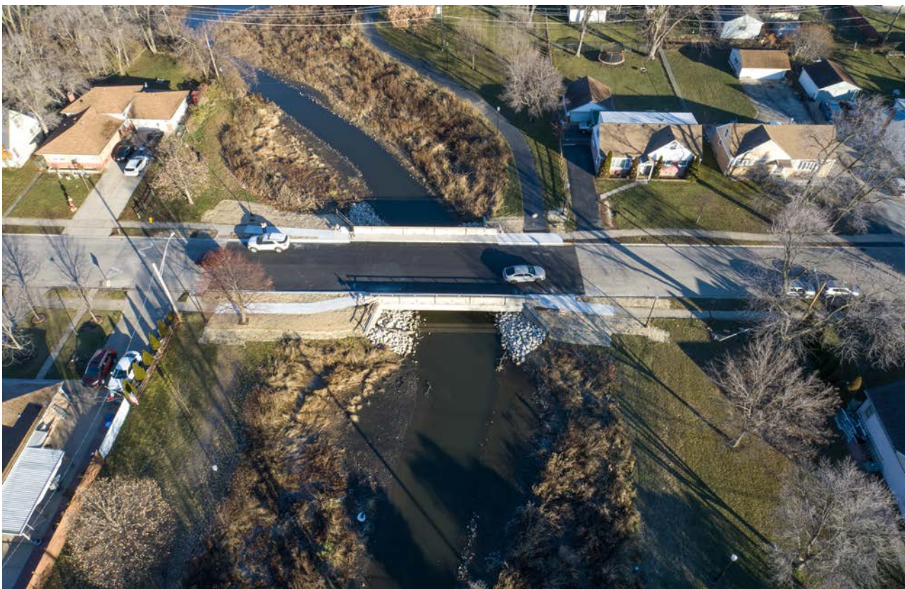
Addison Creek Channel project is designed to improve channel conveyance through six municipalities.
