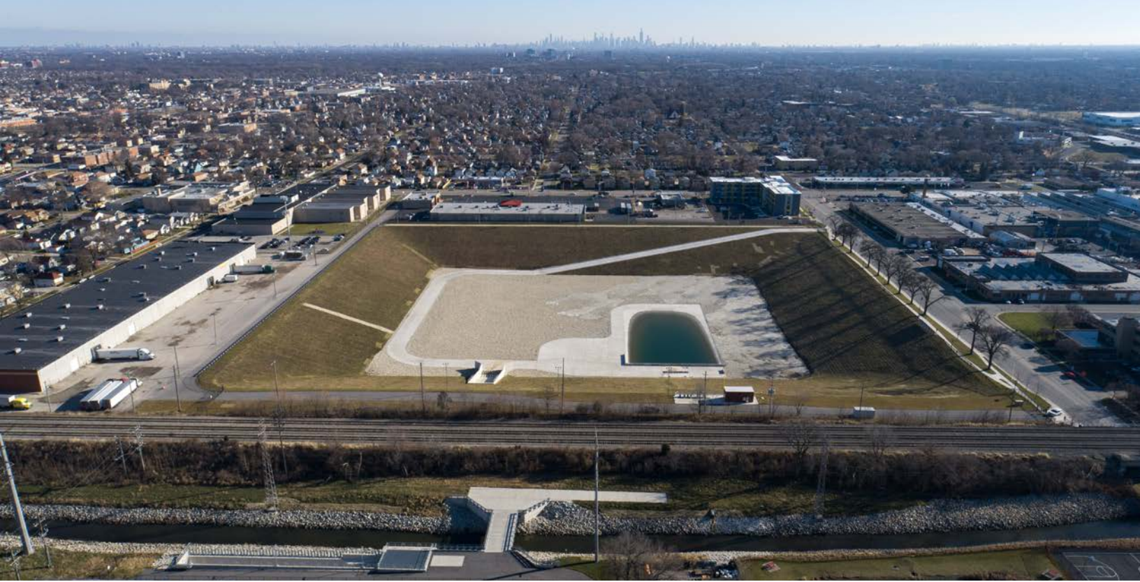
A view to the east showing the Addison Creek Reservoir in Bellwood on Dec. 12, 2023. The Addison Creek Reservoir and the Addison Creek Channel Improvements are two connected flood control projects that will work together to significantly benefit communities along Addison Creek, including Bellwood, Northlake, Stone Park, Melrose Park, Westchester and Broadview. The 600-acre-foot Addison Creek Reservoir will hold 195 million gallons of storage capacity and connect with the Addison Creek Channel to protect the communities from overbank flooding.
