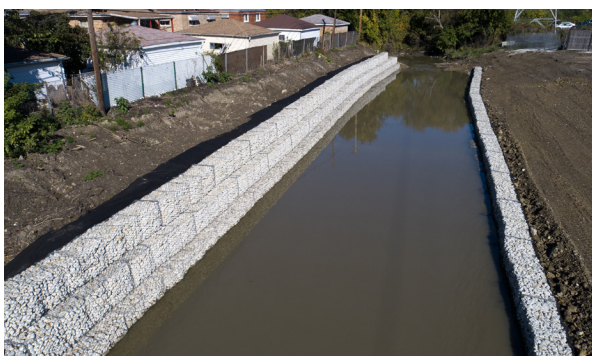
Channel improvements , which clear and widen streams to improve water flow and prevent erosion.
