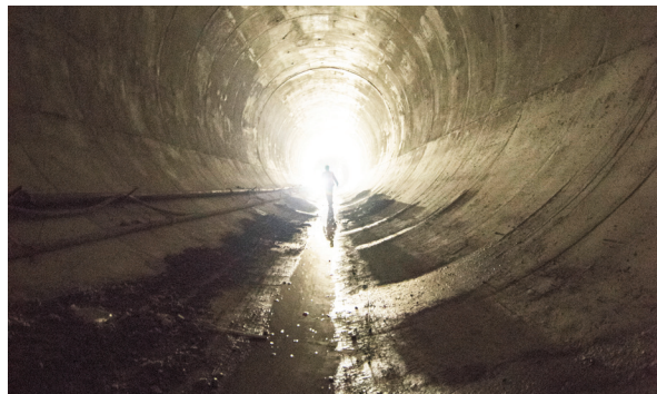
Tunnel and Reservoir Plan (TARP) captures sewage and stormwater during heavy rains to prevent sewer overflows, holding water until it can be treated.
