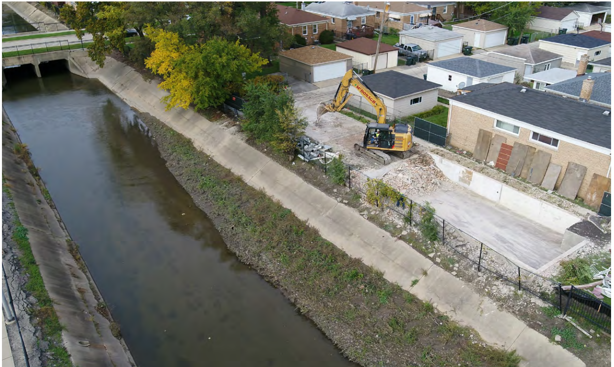
ABOVE A demolition crew removes a home that repeatedly flooded and creates a passive space. Through the MWRD's Voluntary Flood Prone Property Acquisition Program, the MWRD helps local governments pay for the voluntary acquisition of flood-prone property in Cook County.
