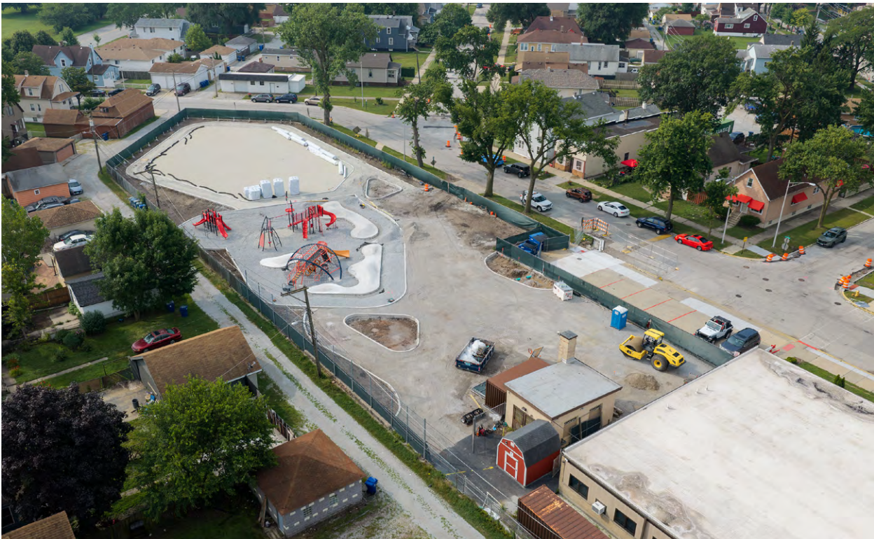
BELOW Construction continues at Burnham Elementary in south suburban Burnham, Ill., as part of the MWRD's suburban green schoolyard pilot program, July 20, 2026.
