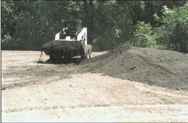
Photograph 1. Biosolids spreaded with Bobcat loader
