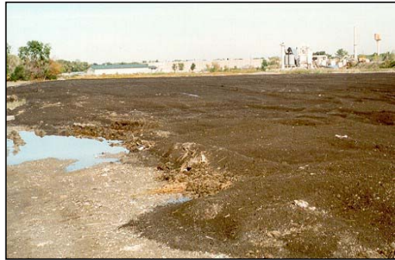
Photograph 2. Biosolids spread over fill before incorporation.
