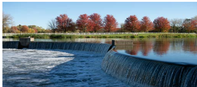
One of five MWRD-built Sidestream Elevated Pool Aeration stations (SEPA), SEPA 4 is stationed in Worth within a 12.5-acre park that attracts many visitors for photo opportunities for weddings, proms, family reunions, and other gatherings. Three five-foot waterfalls add oxygen to 310 million gallons of water every day.
