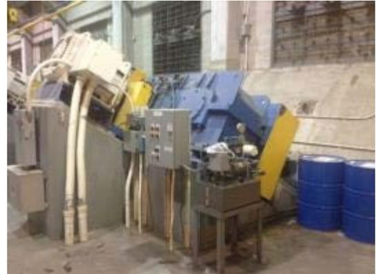
**Project Description** This project will furnish, deliver, and install a replacement gearbox and associated upper and lower bearing for Sidestream Elevated Pool Aeration (SEPA) Stations #2, #3, #4, and #5 in the Calumet Service Area. This project is the Phase II portion of project 20-801-31.
