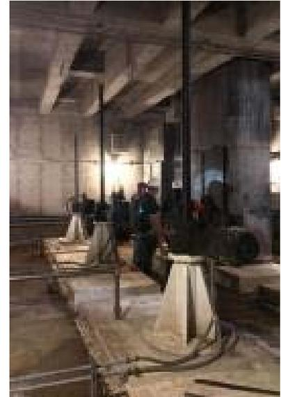
**Project Description** This project entails removing hydraulic gates at the Stickney WRP. Influent control structures M-13-1 and M-14-1 have hydraulic-operated gates in series with motor-operated gates. Hydraulic-operated gates E and F in structure M-13-1 have failed in the closed position, thus reducing operational flexibility during a wet-weather event.
