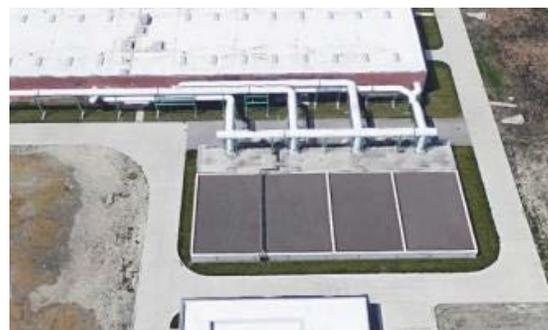
**Project Description** This project entails the construction of three biofilter facilities (one for sludge concentration and overhead weir, one for the southwest coarse screen, and one for the post-centrifuge building). The facilities will include new biofilters, heating, ventilation and air conditioning equipment, ductwork and other ancillary equipment.
