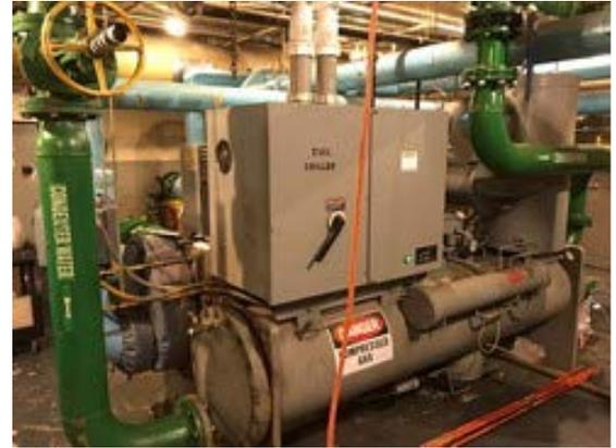
**Project Description** The project entails removing and replacing one 23XL Carrier chiller unit at the Main Office Building. The new unit must be energy efficient, use less harmful refrigerant, and be tied into the building automation system.
