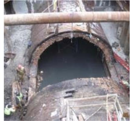
**Project Description** This project will rehabilitate over 100-year-old conduit lying under 39th Street (Pershing Road), stretching from a former pumping station near Lake Michigan to its discharge at the Racine Avenue Pumping Station. The project includes rehabilitation of approximately 15,440 feet of 20-foot diameter brick-lined intercepting sewer and associated manholes and sewer connections.
