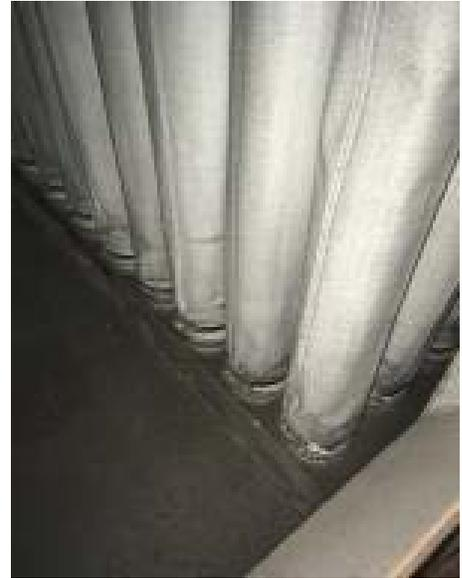
**Project Description** Furnish, deliver, and install primary filter bags in the pump and blower baghouses at the Calumet WRP. The contractor shall install new primary filter bags in 20 baghouses at the Calumet WRP.
