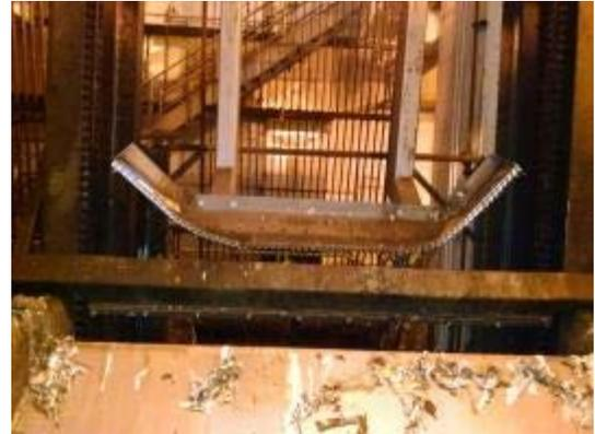
**Project Description** This project entails the removal of existing climber-style southwest coarse screens at the Stickney WRP and the installation of new chain and sprocket-style coarse screens.
