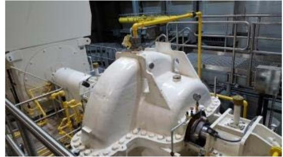
**Project Description** The project entails rehabilitating the suction and discharge valves in the main sewage pumps at the Calumet Tunnel and Reservoir Plan (TARP), which includes integrating the medium voltage drive auxiliary chillers into the house-chilled water system, balancing and aligning rotating assemblies, and upgrading obsolete prime-mover vibration and temperature monitoring systems.
