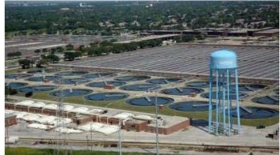
**Project Description** The city water tank at the O'Brien Water Reclamation Plant has sustained corrosion and is only equipped with a temporary cover. Under this project, the tank will be re-coated inside and out, and a permanent cover will be installed. The Stickney city water tank, erected in 1958, was last rehabilitated in 1996. Rehabilitation of the water tower will include all necessary structural improvements.
