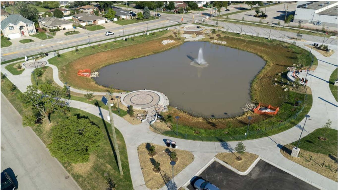
*The District partnered with the Village of Niles to construct a relief storm sewer and surface and underground stormwater storage areas near Greenwood Avenue to provide flood relief to nearby homes and businesses. The project has the capacity to store and detain more than 4.5 million gallons of stormwater to help mitigate flooding in Niles.*
