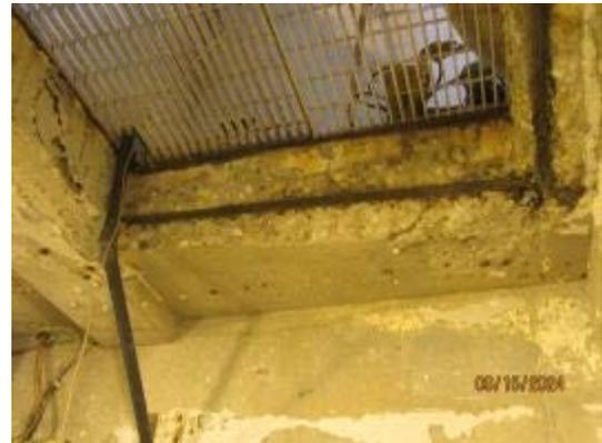
**Project Description** The existing concrete at the Walters Road Pumping Station within the wet well area is cracked and spalling along the floors and ceiling slabs. Removal of concrete debris, filling existing cracks, and leveling is required to restore the structural integrity of the wet well.
