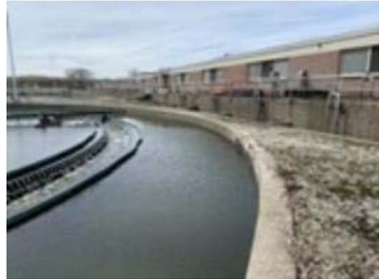
**Project Description** This project entails concrete rehabilitation and the installation of railing at the Battery A final settling tanks and influent channels, air piping replacement in the Battery A aeration tanks, and the installation of mechanical mixers in the Battery B aeration tanks at the Stickney WRP. This project also includes the installation of a transfer slab below "F" Street to protect the Battery A main effluent conduit below and allow heavy traffic over the road.
