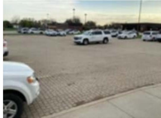
**Project Description** This project will restore the permeable pavement parking lot at the Stickney WRP, which includes replacing stone joint material, cracked or damaged pavers, and leveling as needed.
