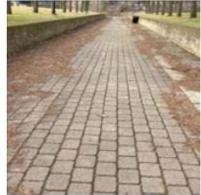
**Project Description** This project entails removing, salvaging, re-leveling, and re-installing pavers to create a walkway surface that is substantially compliant with recommendations articulated in the Americans with Disabilities Act.
