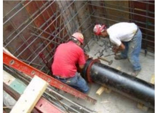
**Project Description** This project will replace Section 1 of the existing North Side Sludge Pipeline with 19,000 feet of 20-inch diameter force main, construct air relief, blow off and clean out structures, and rehabilitate 43 existing structures located in the City of Chicago and the Villages of Lincolnwood and Skokie.
