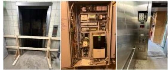
**Project Description** This project entails modernizing the east and west Tunnel and Reservoir Plan elevator controls at the Calumet WRP and rehabilitating the north vent elevator at the Mainstream Pumping Station.
