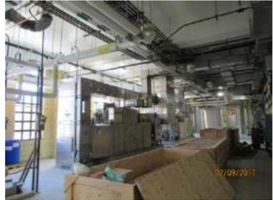
**Project Description** This project will remove ineffective heating, ventilation, and air conditioning (HVAC) equipment servicing the Ultraviolet Building and install effective HVAC, air condenser cooler, and rooftop units. In addition, this project will replace the existing Switchgear Building air handling unit with new effective rooftop air handling units that are air condenser cooled.
