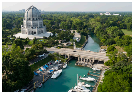
Wilmette Pumping Station
