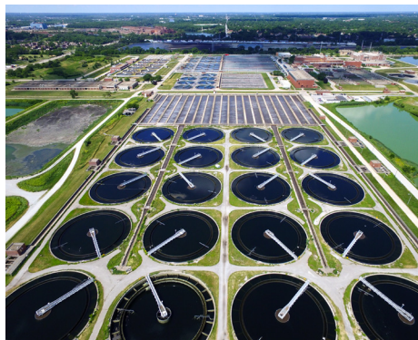
Calumet Water Reclamation Plant
