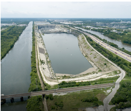
McCook TARP Reservoir
