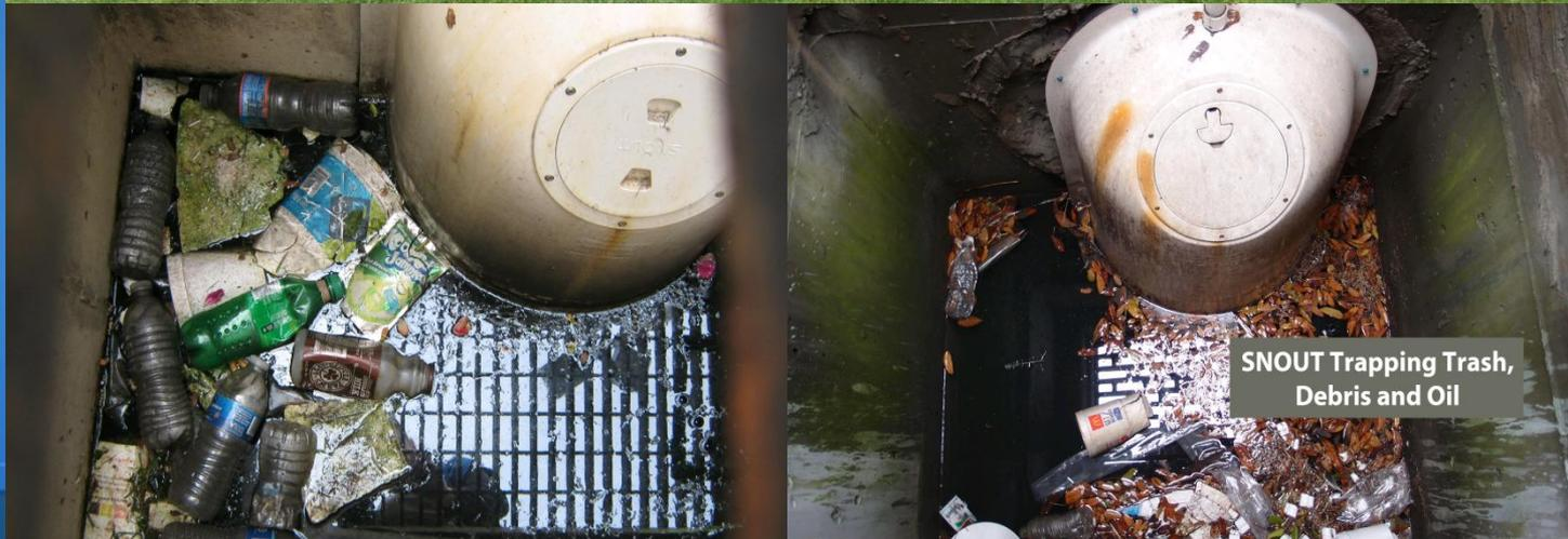
SNOUT Trapping Trash, Debris and Oil
