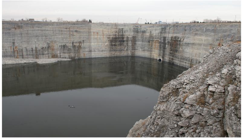
*Completed in 2015, Thornton Composite Reservoir has a storage capacity of 7.9 BG and is the largest combined sewer reservoir in the world. The reservoir, with a surface area of approximately 83 acres, serves a 90-square-mile area in Cook County. The reservoir provides an estimated \$40 million per year in flood control benefits to 556,000 people in 14 communities, including the South Side of Chicago and 13 suburban communities.*
