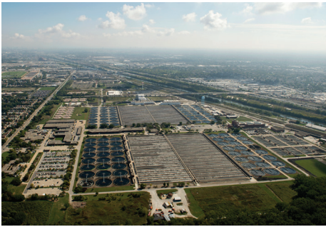
Stickney Water Reclamation Plant with the Chicago Sanitary and Ship Canal
