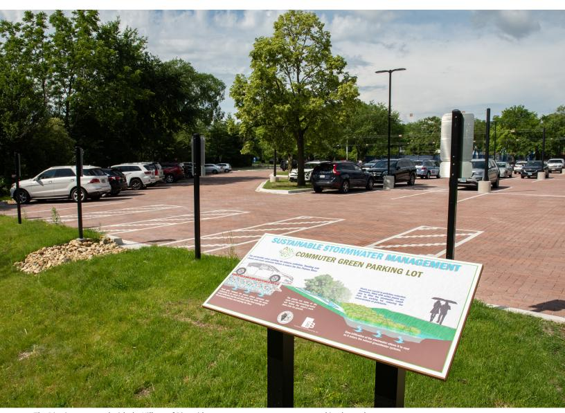
The District partnered with the Village of Riverside to construct a new commuter parking lot and bioretention area that will provide parking for Metra commuters and more than 237,000 gallons of stormwater storage per rain event. The permeable parking lot and rain garden will reduce the current load to the combined sewer system and help alleviate flooding within the project area.
