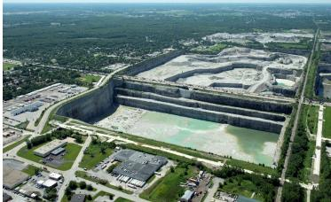
*Left*: The world's largest reservoir, the Thornton Composite Reservoir, can hold 7.9 billion gallons of water emanating from the tunnels on the east wall.
