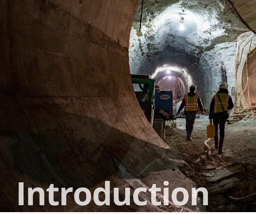
The TARP System's tunnel segments add up to more than 110 miles of storage capacity traversing about 300 feet below Chicago area waterways. The tunnels are designed to store more than 2.3 billion gallons of water in segments that are as large as 33 feet in diameter. TARP helps protect Lake Michigan and area waterways from pollution by providing an outlet for combined sewer overflows, while also mitigating street and basement backup flooding.
